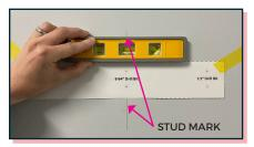
Locate stud within the wall you intend to hang your Reflect and mark with a pencil. Level and tape wall mount template with middle two cross marks centered over stud mark.
