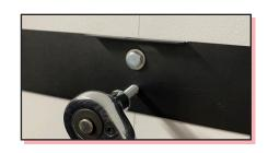
7. Drive in the two lag screws into the pre-drilled pilot holes.
