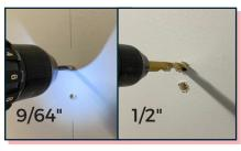
Using a 9/64" drill bit, drill two pilot holes for the lag screws.
